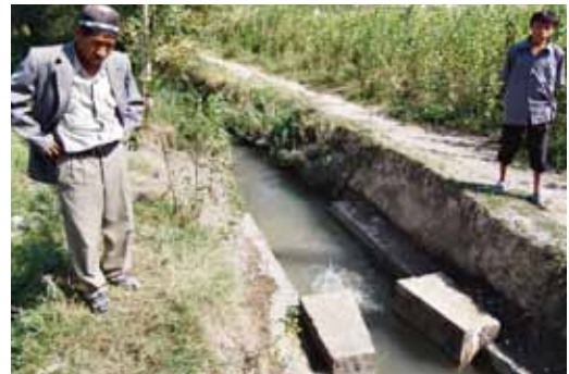
Sustainable water management in Central Asia: In the area covered by the project, savings on up to 30% of the agricultural requirement for water were achieved
