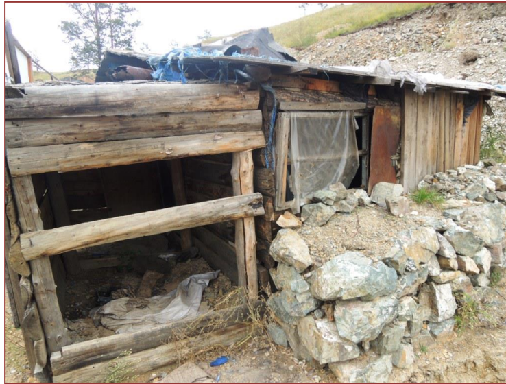
Figure 2. Mine entrance at the Budanch hard rock mine site
