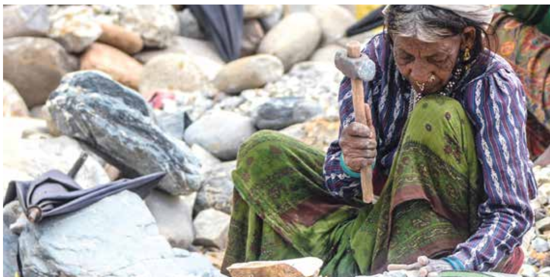
Crushing stones for bridge construction. Pramad Bhattarai
